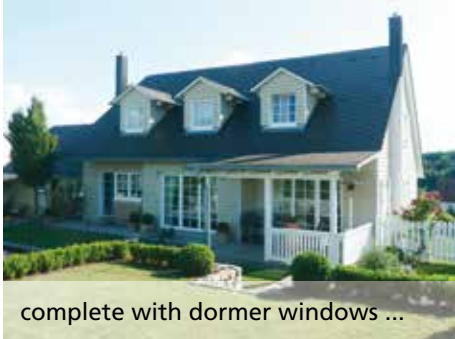
Rafter and purlin construction ...
