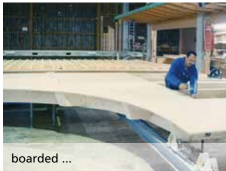
joints finished on tectofix 3000 ...
